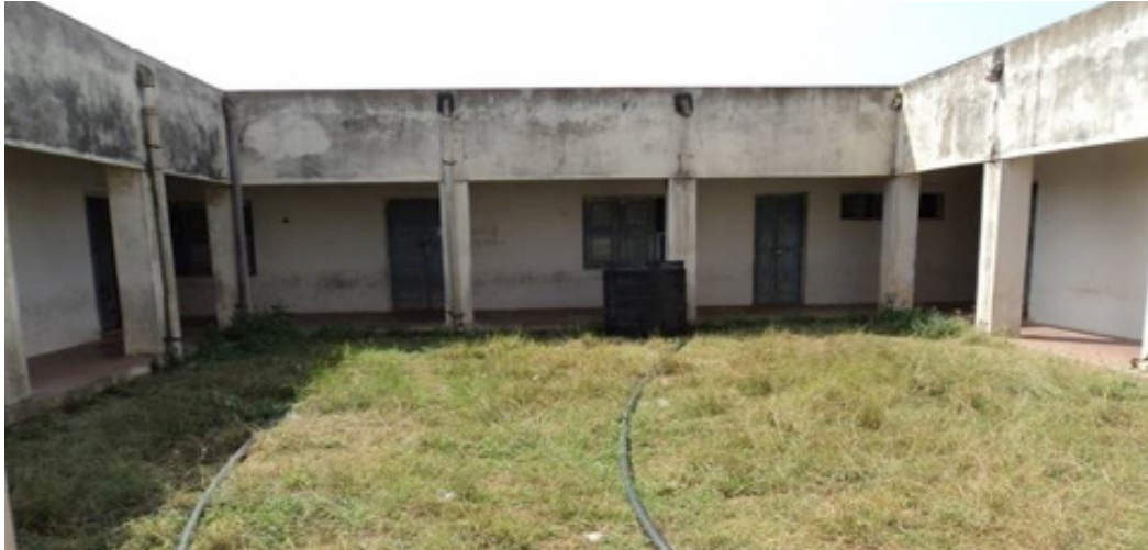
TDC before renovation
