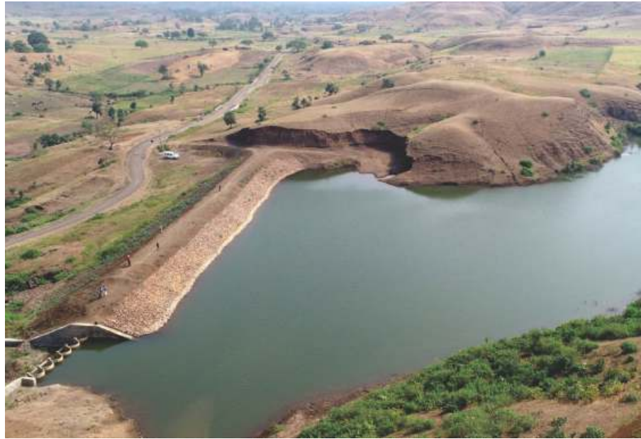
Water harvesting structure created by the people of Jod Mohra, Madhya Pradesh, with Reliance Foundation's support.
